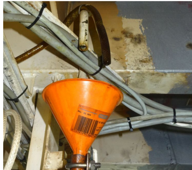
Picture 16 - self-made rubber hose constructions...
