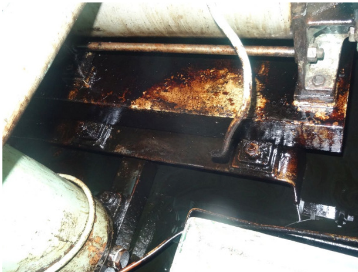
Picture 20 - HFO spill in engine room
