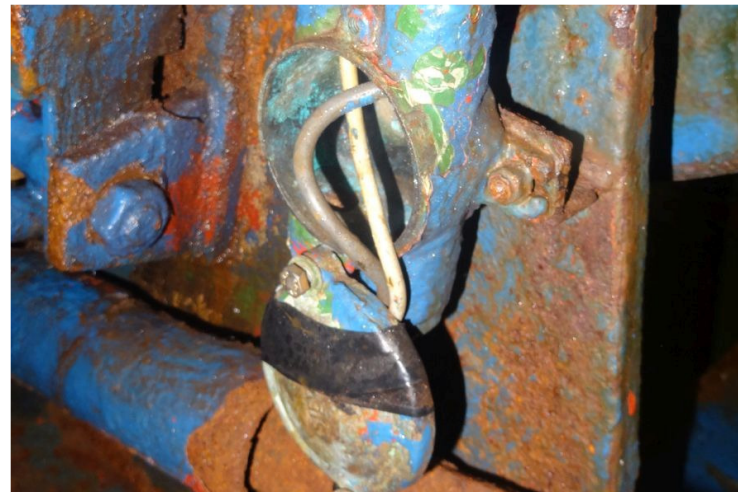
Picture 11 - electric installations on deck ...
